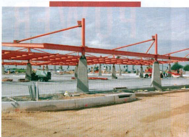
Closer view of supports for covered parking.
