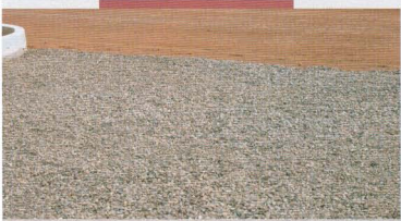
A section of rock sub-base ready to have pervious concrete poured onto it.
